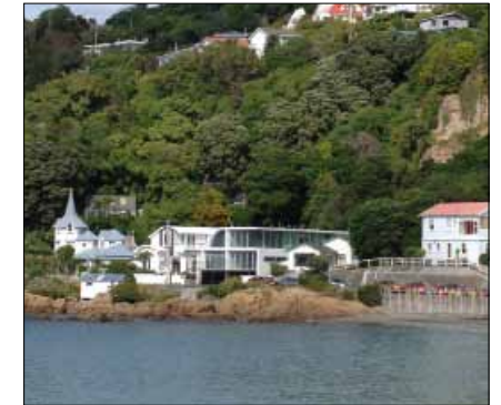
As Built View
